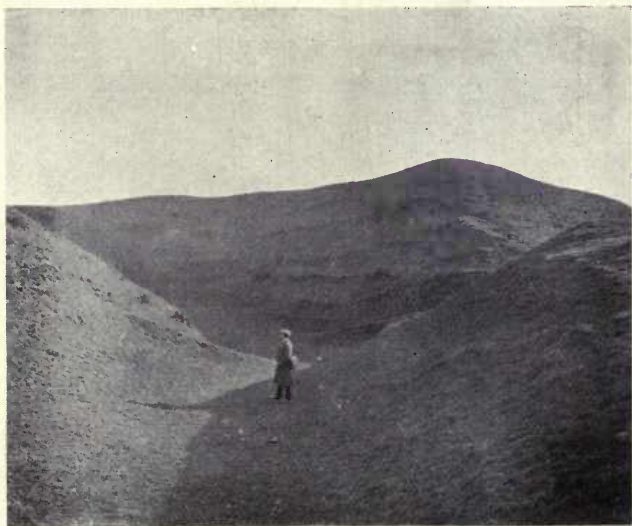
Earthworks, Builth Castle
